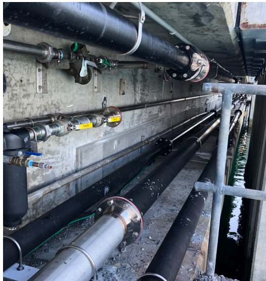
PHOTOS: Top - Given the highly corrosive nature of the Wharf new piping had to be installed. This is the finished fire protection riser. Bottom - Replacement of all corroded cast iron piping was done on the wharf face utilizing stainless steel utility connection risers and valve.
